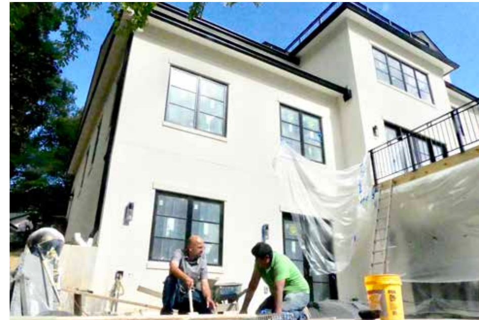
Resit supervising Garfield construction
